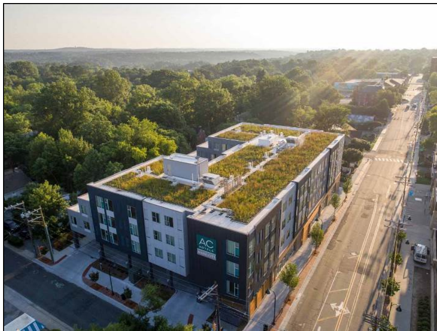
Figure 11: Example green roof
